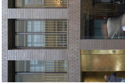
GAA - GOLD ANODISED ALUMINIUM. BALUSTRADES + WINDOW FRAMES
